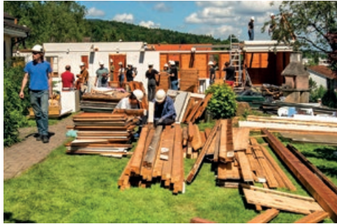
Disassembly of Oetwil am See Music Pavilion for Reuse © Buser Hill Photography, CEA lab
